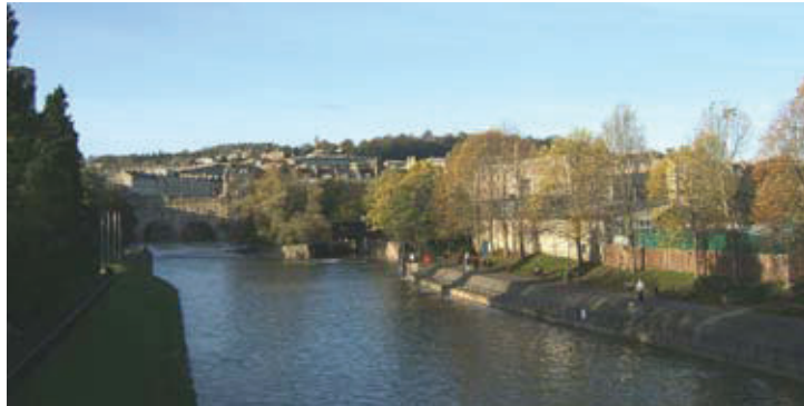
North Parade Bridge towards Pulteney Bridge and Beacon Hill
