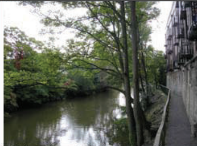
R6 Riverside path at Walcot, Part of the riverside walk which is not currently continuous
